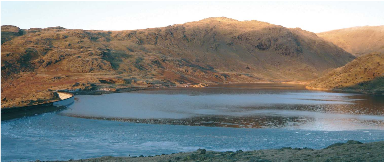
Seathwaite IR after completion of refurbishment
