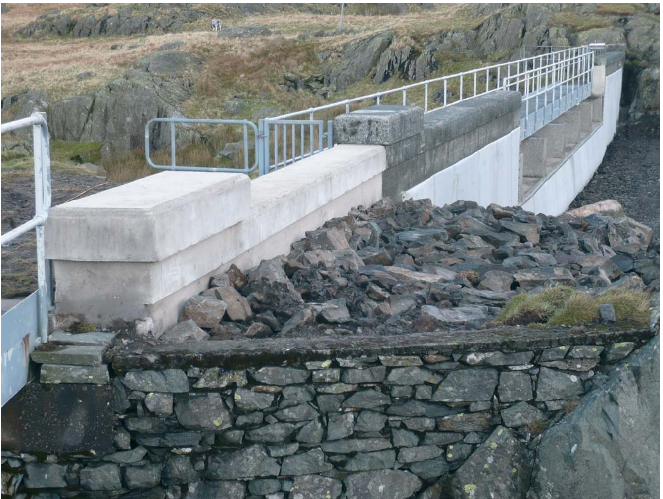
Modifications to auxiliary overflow structure and wave wall extension
