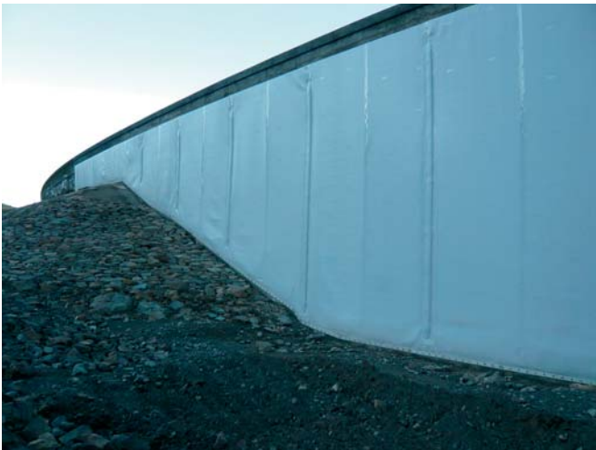
Photos show new membrane on upstream face of concrete dam (left) and auxiliary overflow (right)
