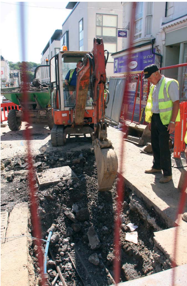
Mains replacement work continues on North Road, Brighton
