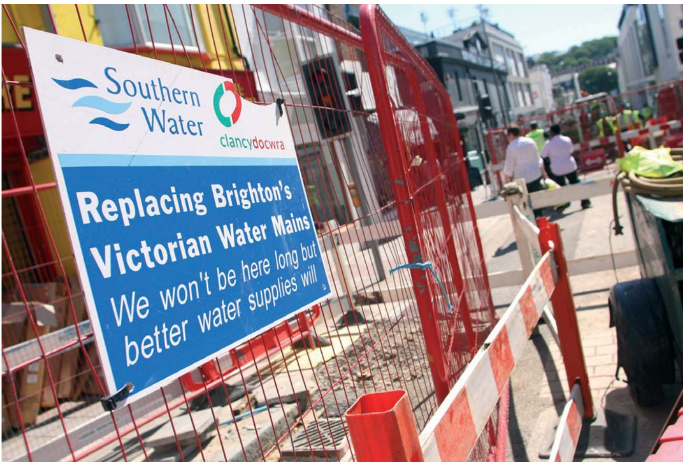
Mains replacement work continues on North Road, Brighton
