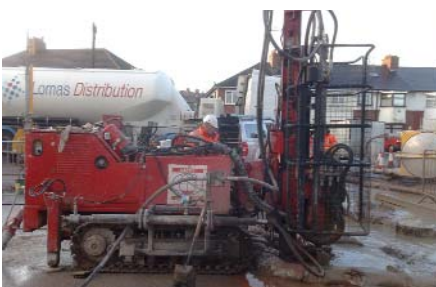
Drilling of Jet Grouted Columns
