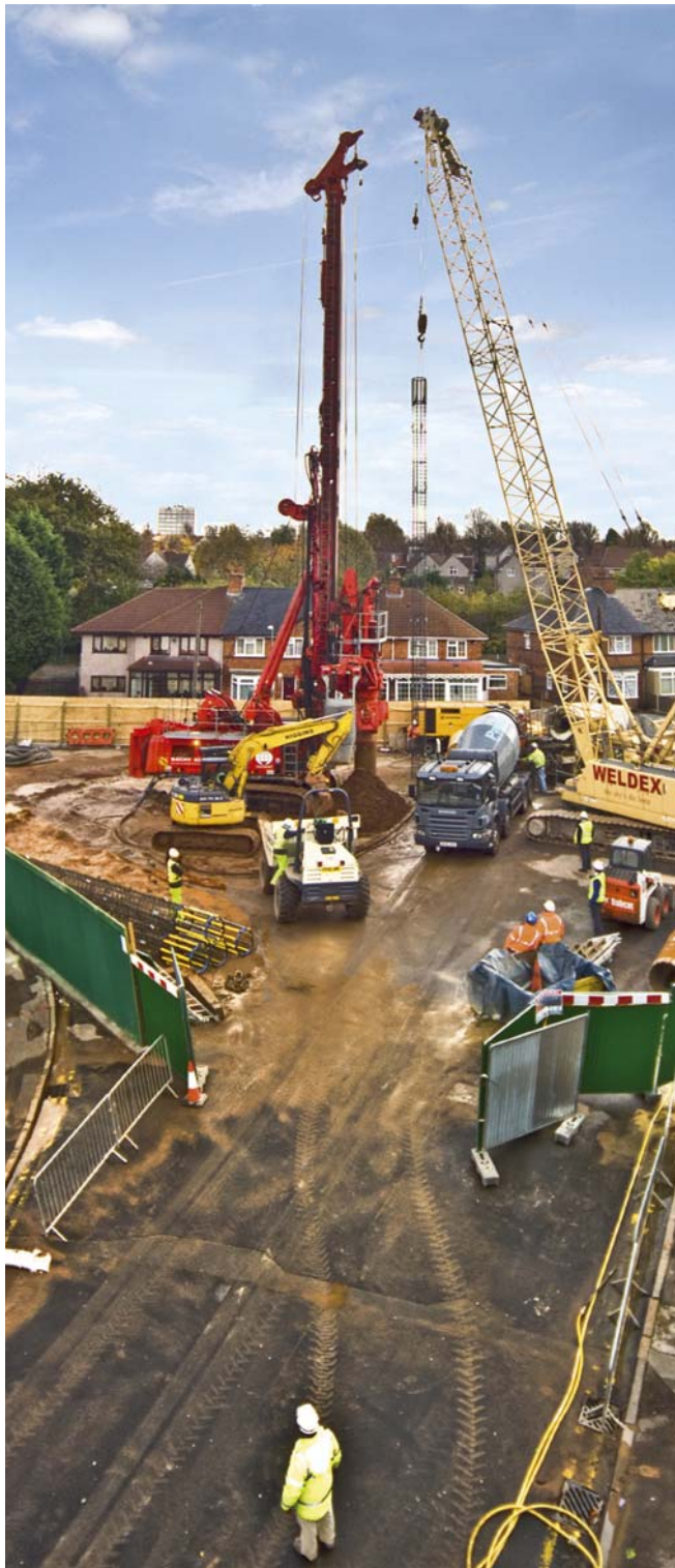
Foxton Road Site during piling works
