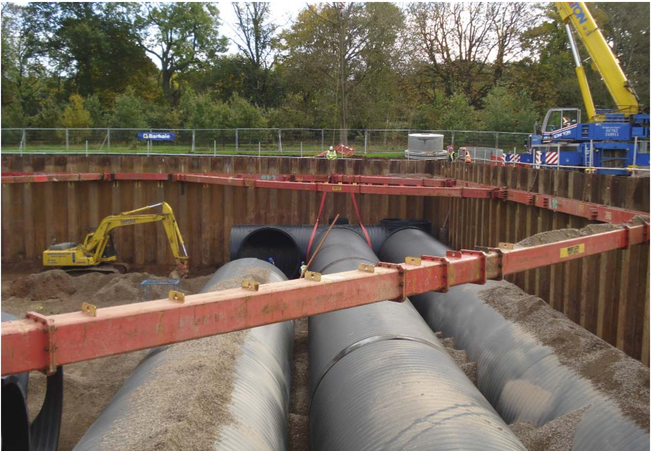
Weholite tank construction
