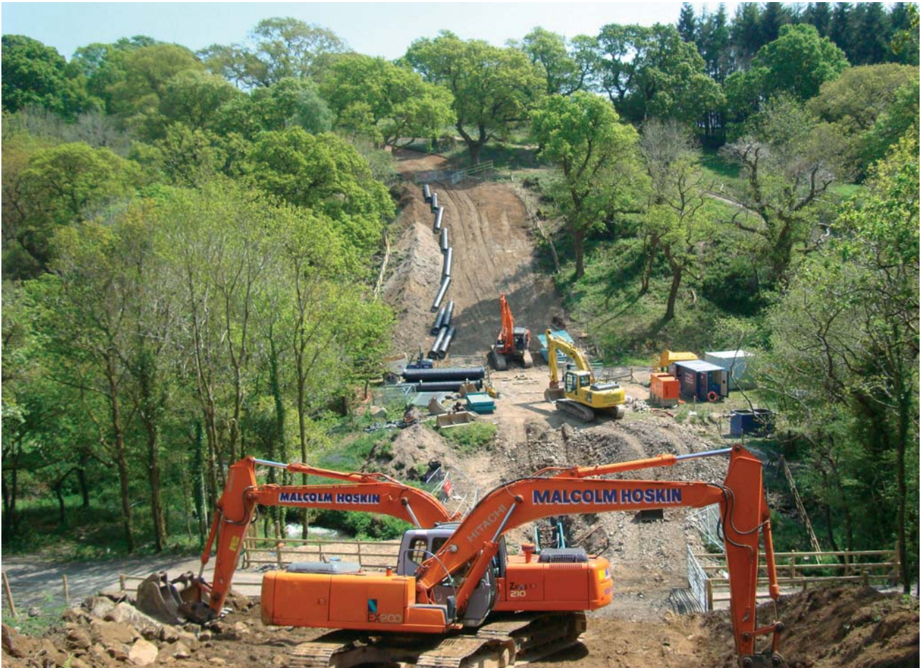
Construction within Newnham Park
