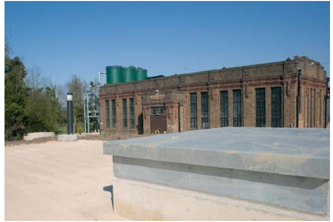
Works completion Photograph by Ady Kerry, courtesy of South East Water
