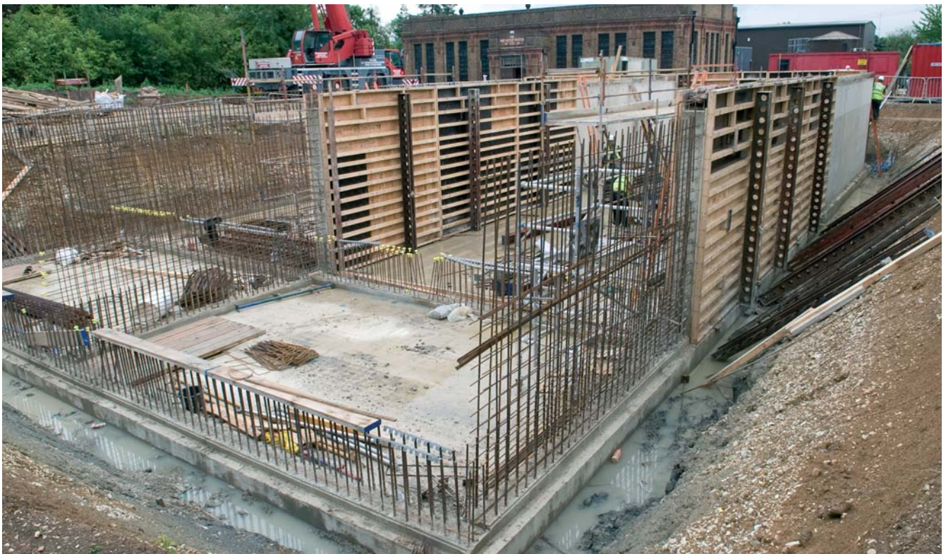
Contact and backwash tanks during construction
