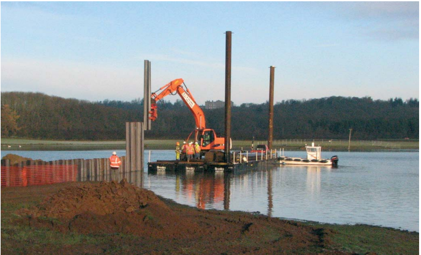
Constructing a “marine” lagoon in Rutland Water
