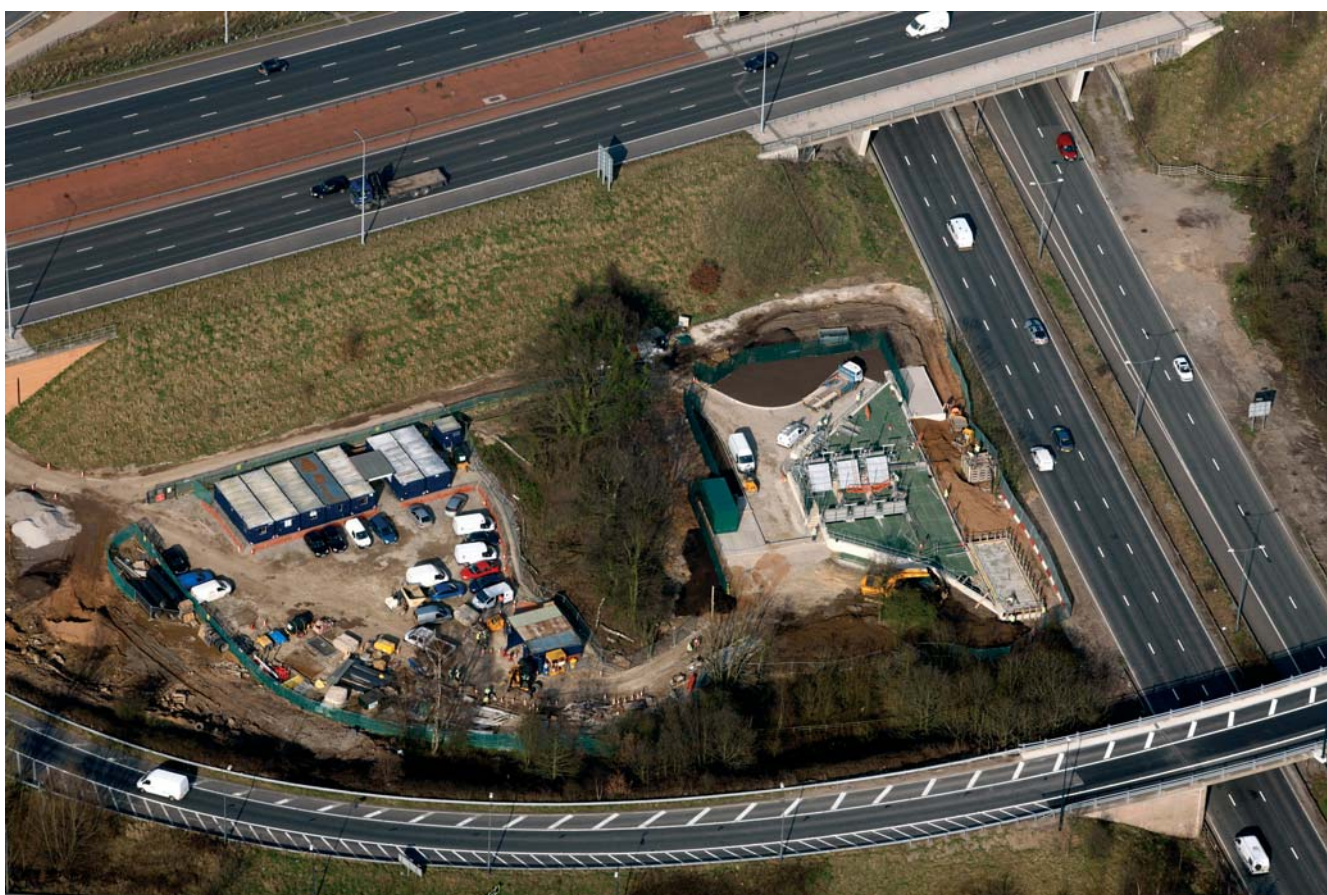
Princess Parkway Screening Chamber
