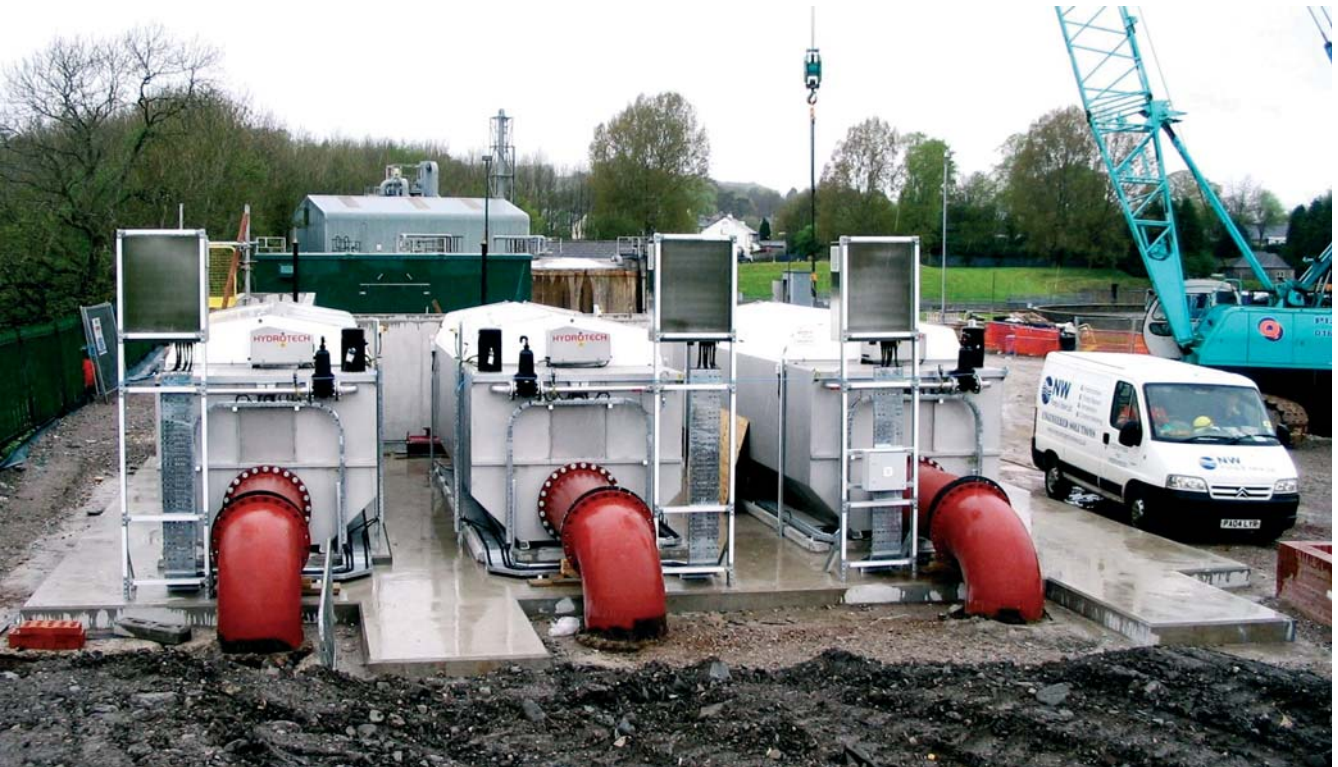
Disc filters during construction, outlet end
