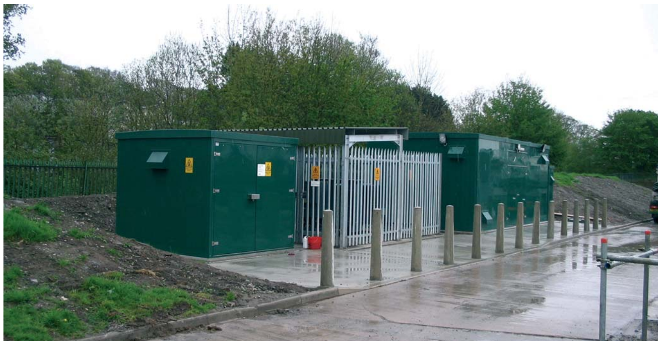
From left, New REC Incomer kiosk, Ring Main unit and new switchboard kiosk
