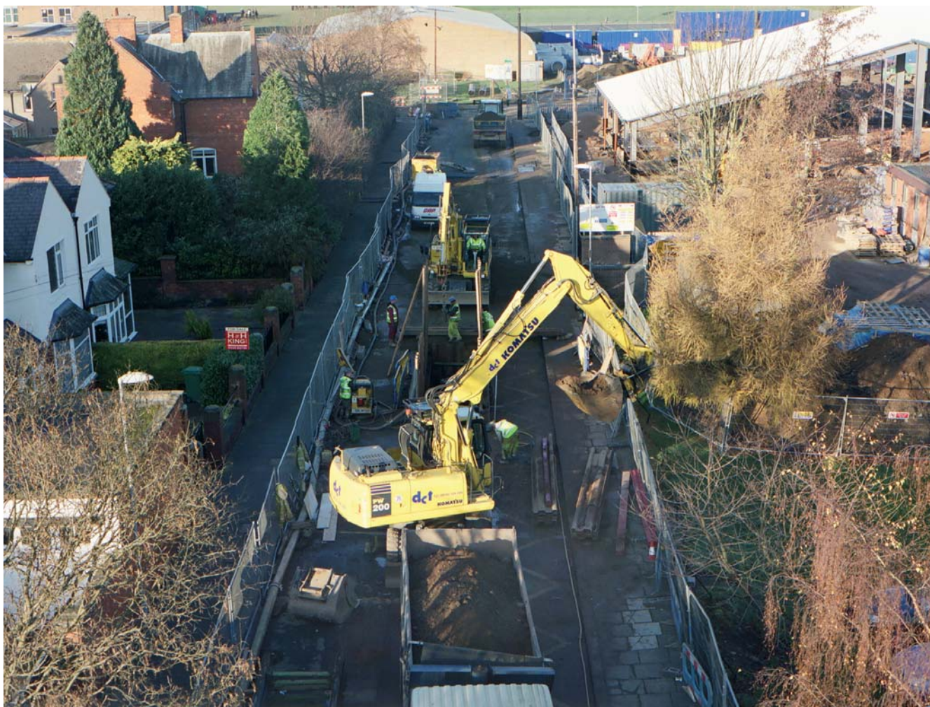
Construction work underway at Lismore Place
