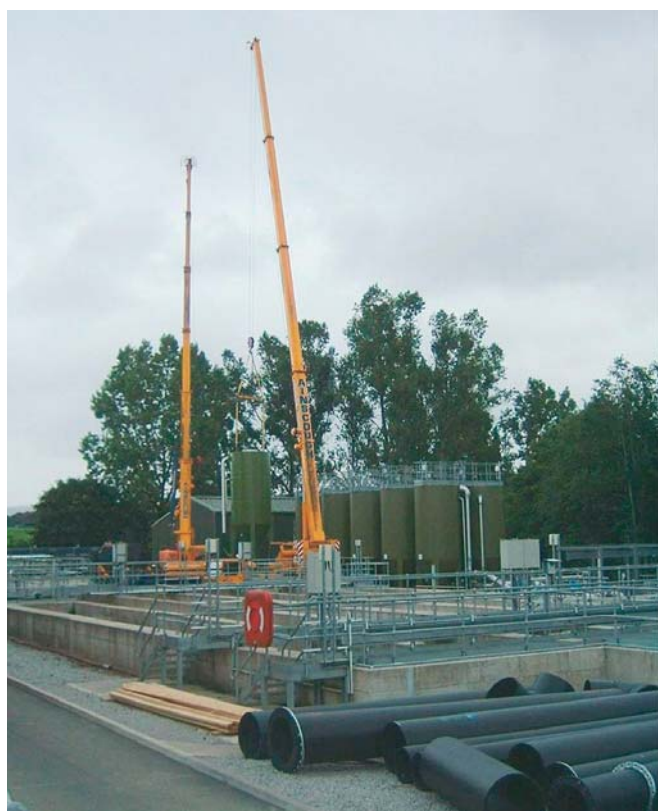
Lifting a new NSF unit into place on the far side of the existing 10 COUF units (left) and offloading 2 new NSF units adjacent to existing 10 COUF units (right)
