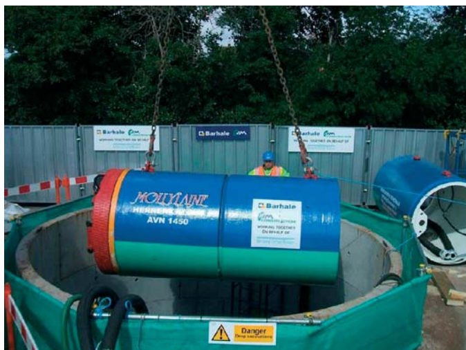
TBM Launch (left) and TBM Jacking (right)
