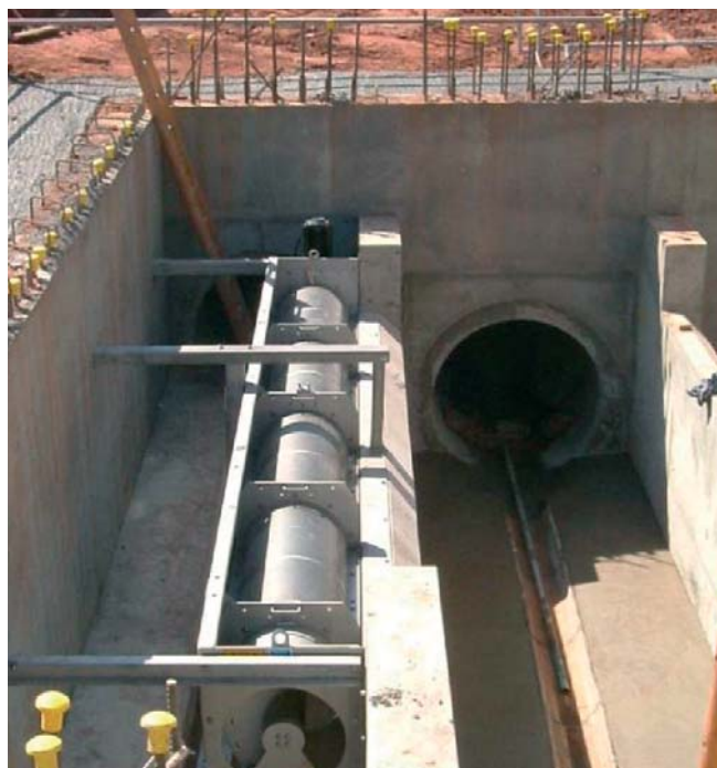
CSO screens installed
