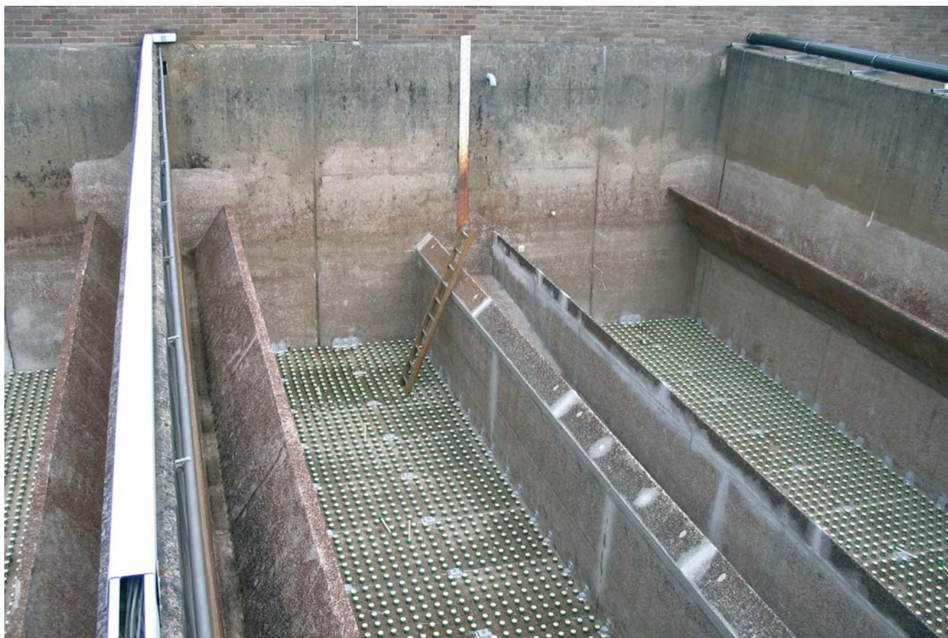
Franklaw WTW: 1st stage filter refurbished with new nozzles, awaiting new filter siphons & GAC
