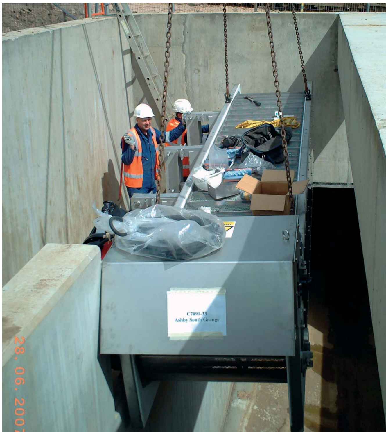
Screen installation at Ashby South Grange
