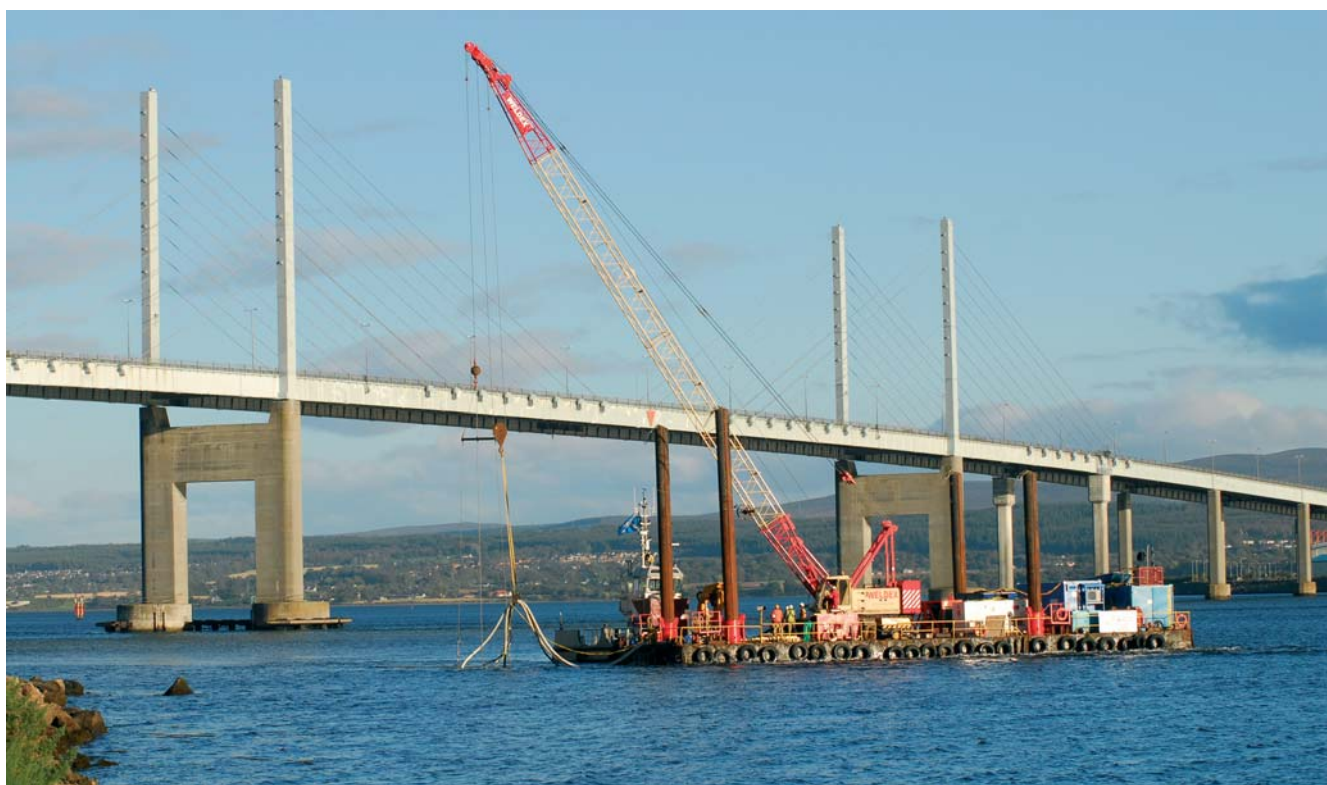
The pipelaying barge next to the Kessock Bridge
