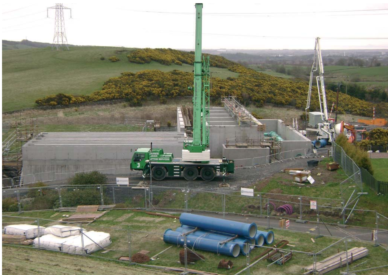
Lomond Hills WTW under construction photo shows inlet & RGF
