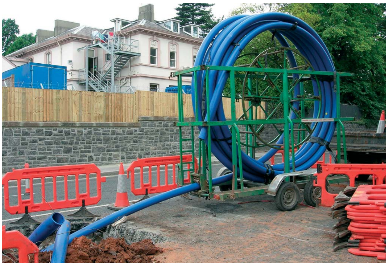
Pipebursting continues in South Belfast
