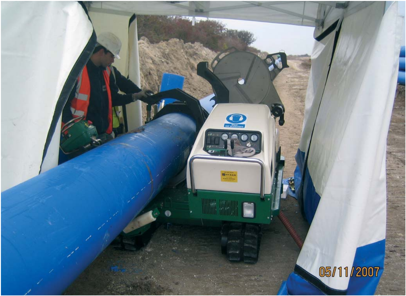
On-site butt fusion welding
