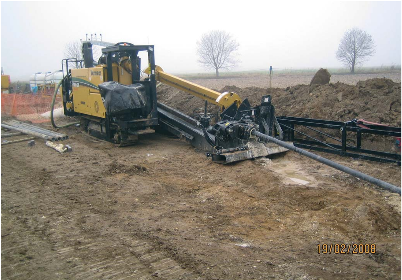
Directional drilling at Lea Brook
