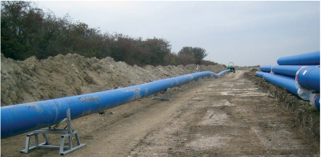
Pipe strung out along the easement
