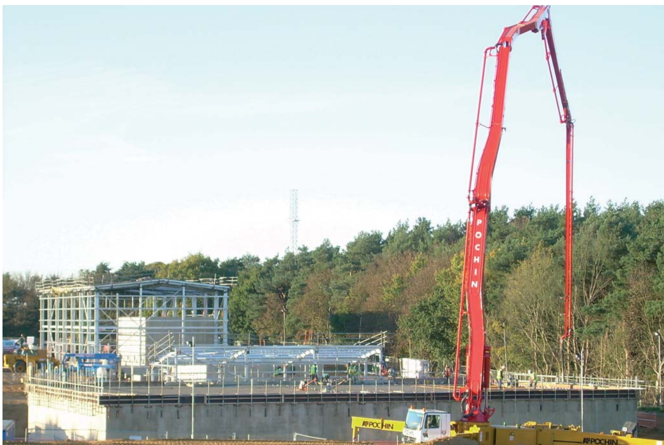
63 metre concrete pump pouring reservoir roof
