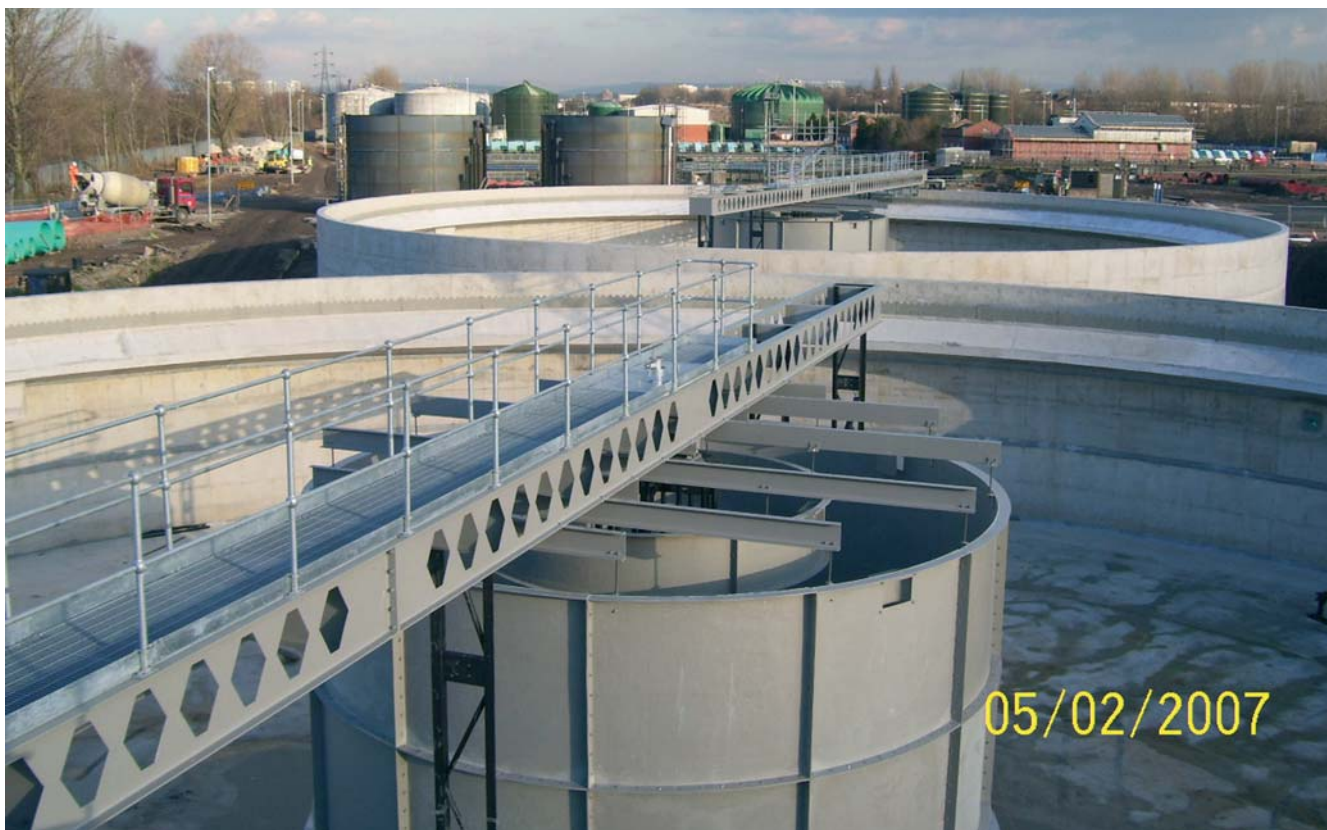
Stockport WwTW: Overview of works
