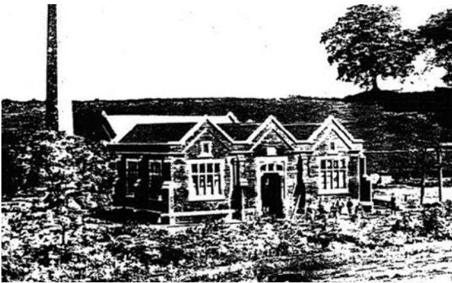
courtesy: Norwest Holst Ltd & Severn Trent Water PLC
