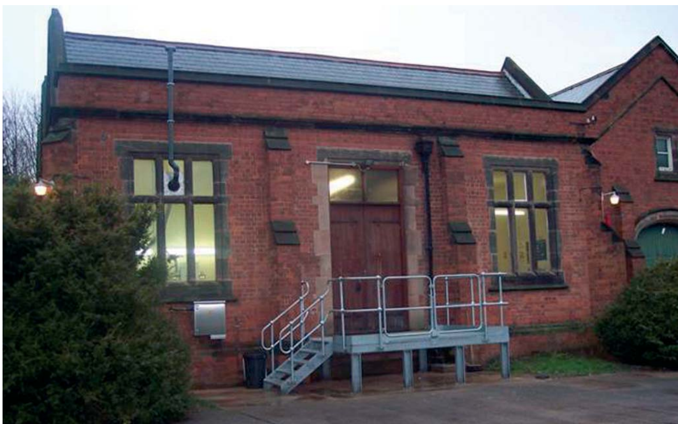
Stanton-by-Bridge Pumping Station first constructed in 1892 & now modernised
