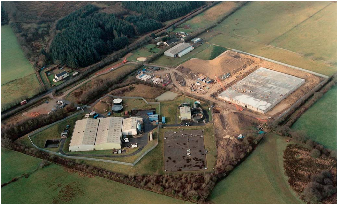
Northcombe New Service Reservoir: under construction & Northcombe WTW
