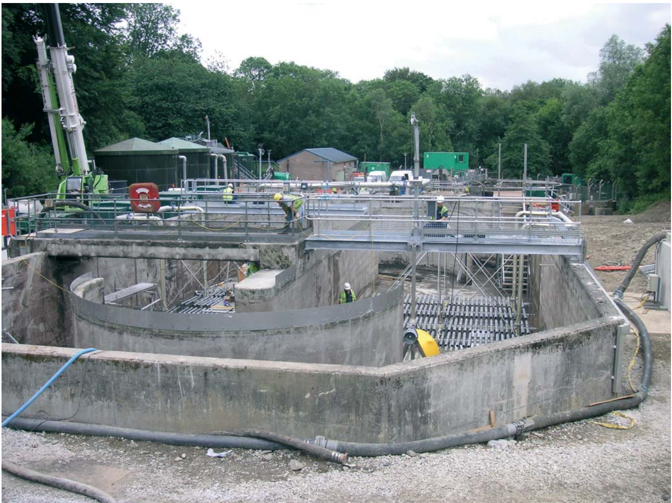
Callington STW under construction
