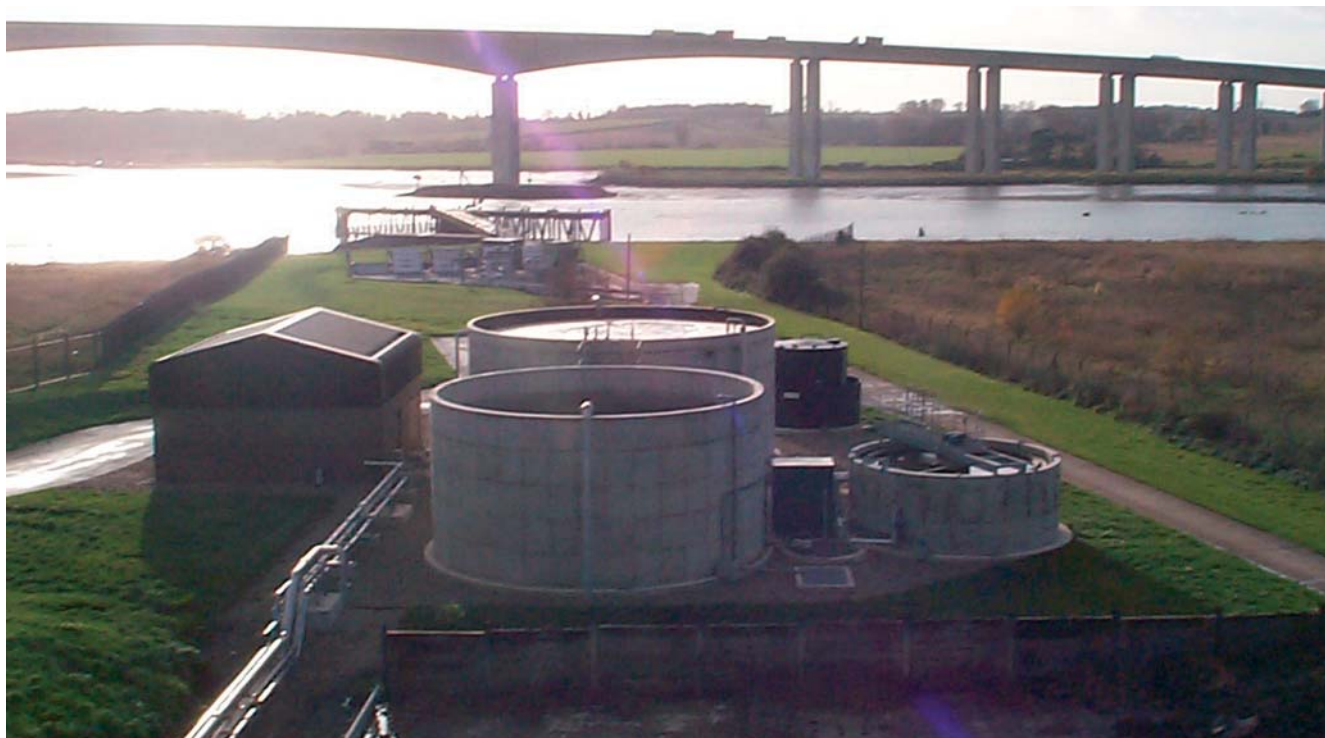
Cliff Quay AMTREAT® Sludge Liquor Treatment Plant
