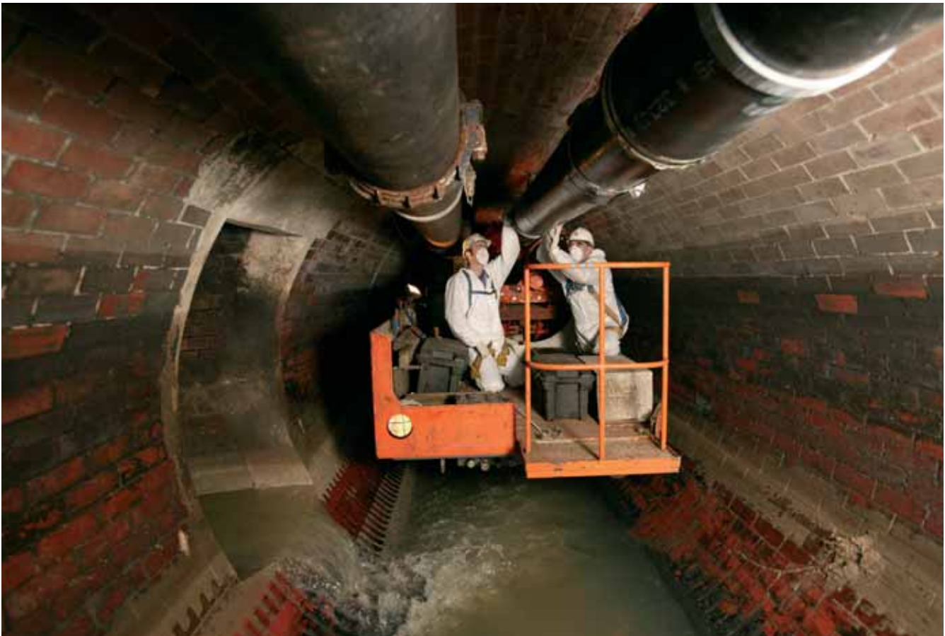
Putting finishing touches to the newly installed piping
