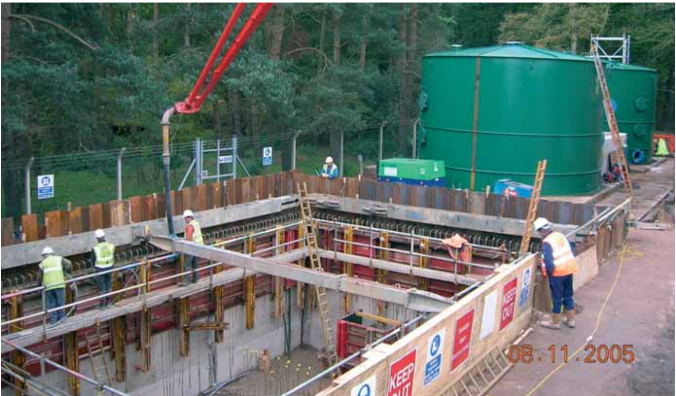
Milford & Bednall: New filters & high lift pumping station under construction
