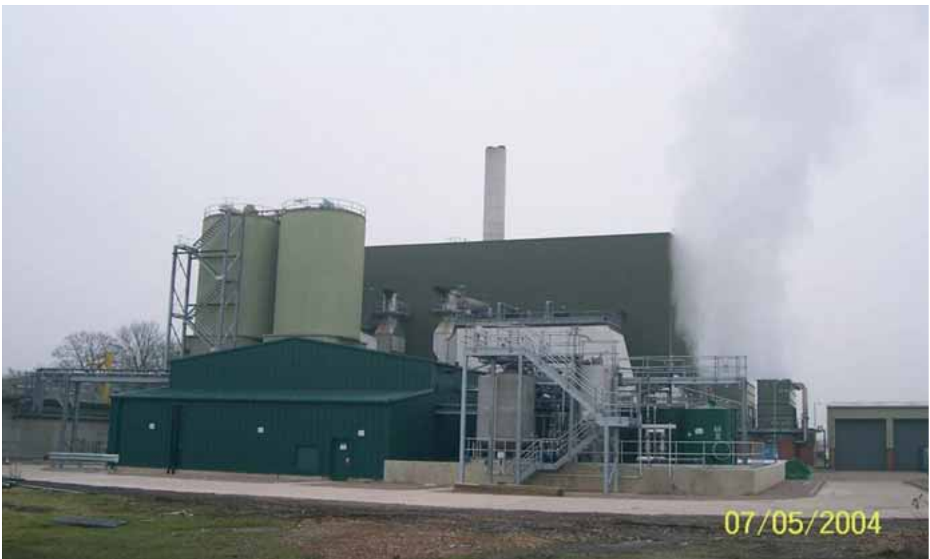
Coleshill Sewage Sludge Incinerator
