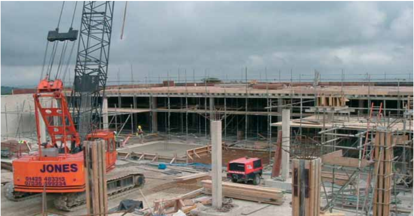
Stanborough: Service reservoir under construction
