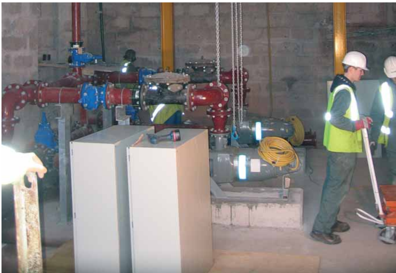
Refurbishment of existing pumping station at Geevor
