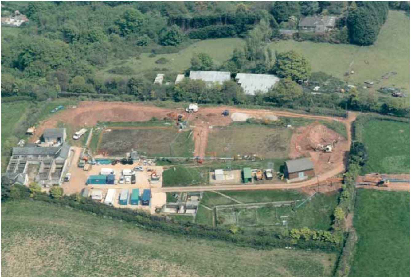
Burrows WTW scheme under construction
