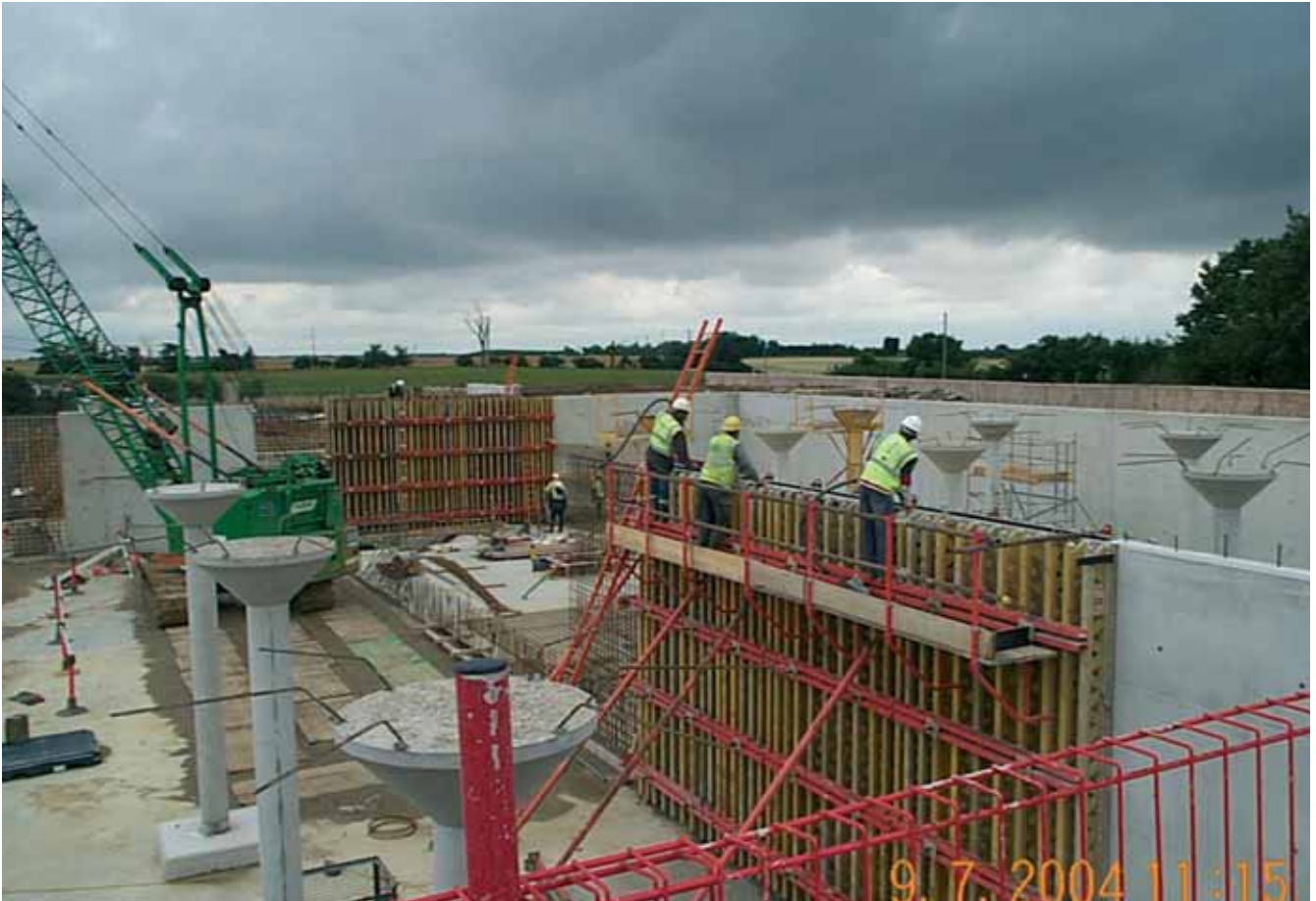
Ford Quality Scheme: New service reservoir under construction
