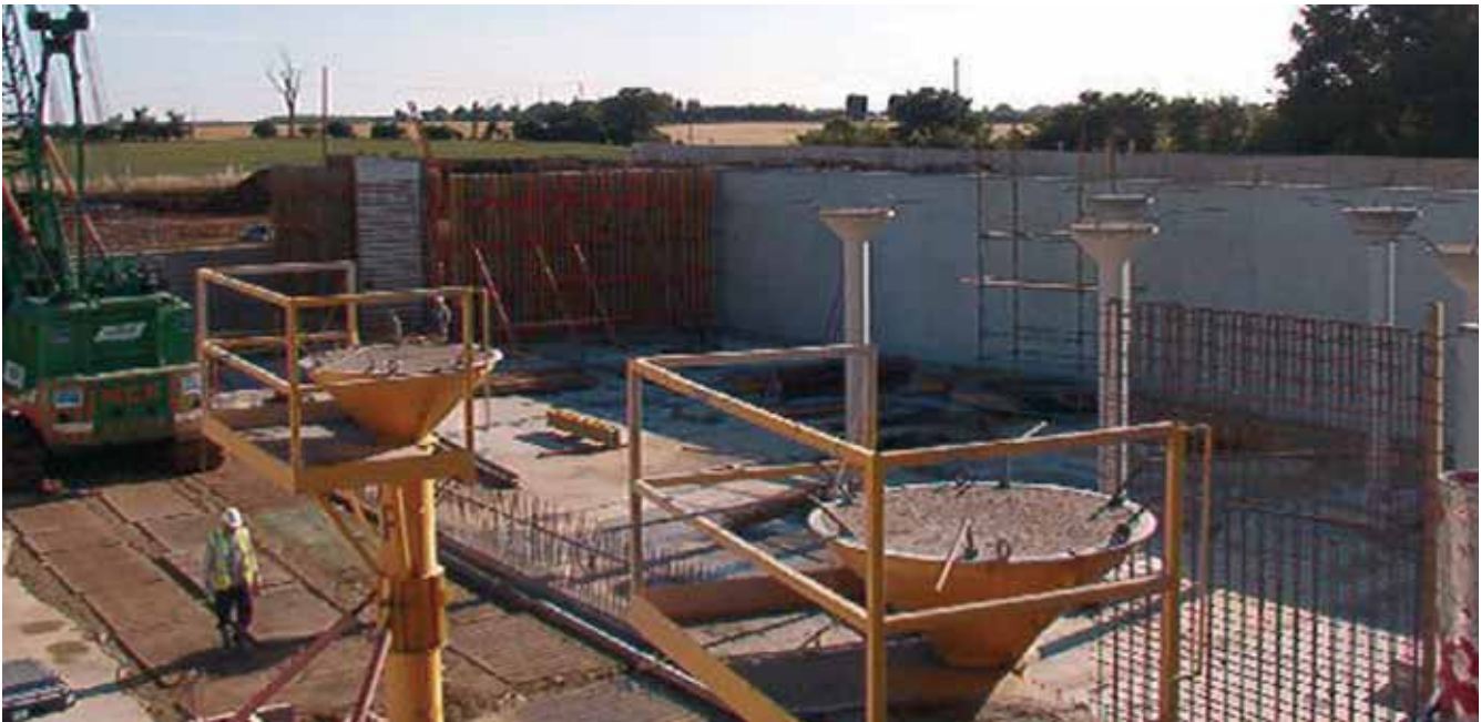
Ford Quality Scheme: under construction
