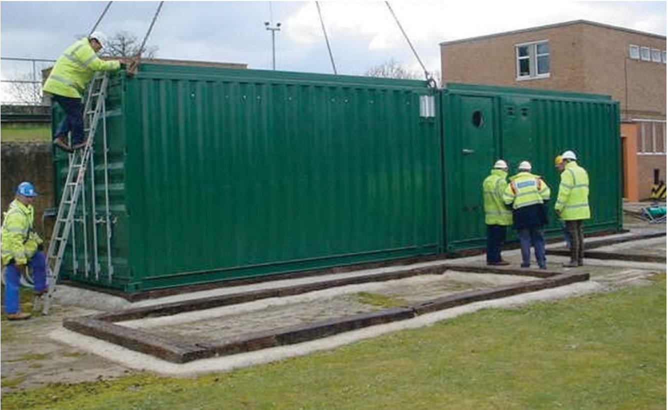
Emergency Pkg Plant unloaded ready to set on base
