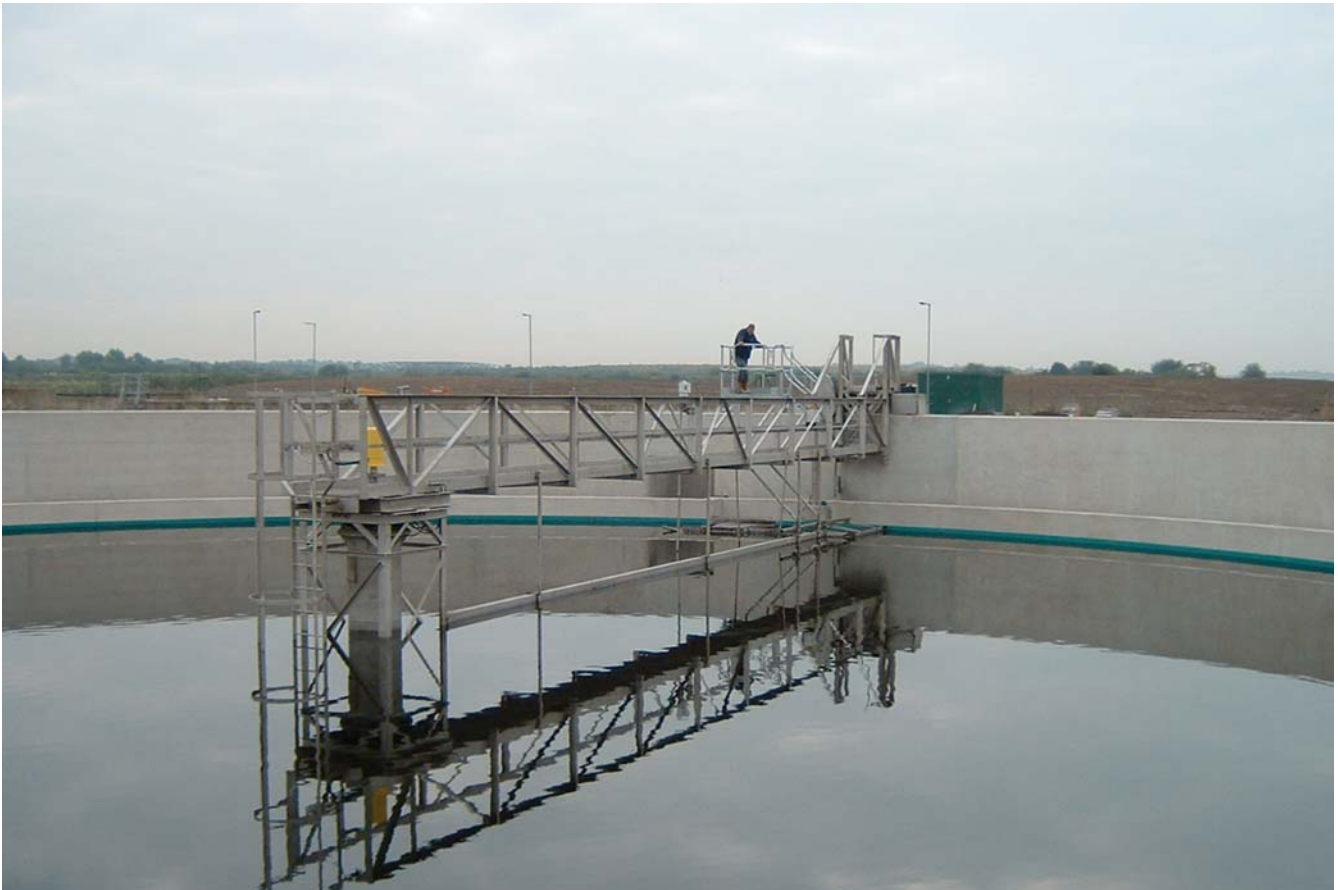
Warrington North WwTW: 35m Rim Flo clarifier – commissioning phase
