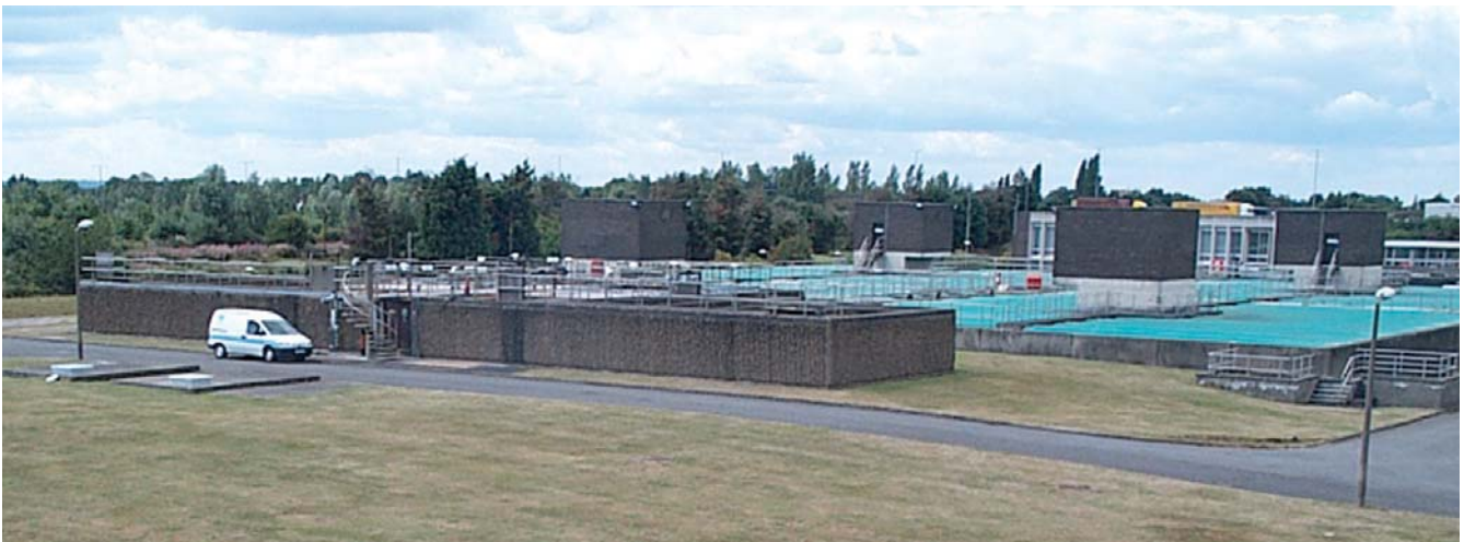
Iver WTW: Preferred location from preozonation building
