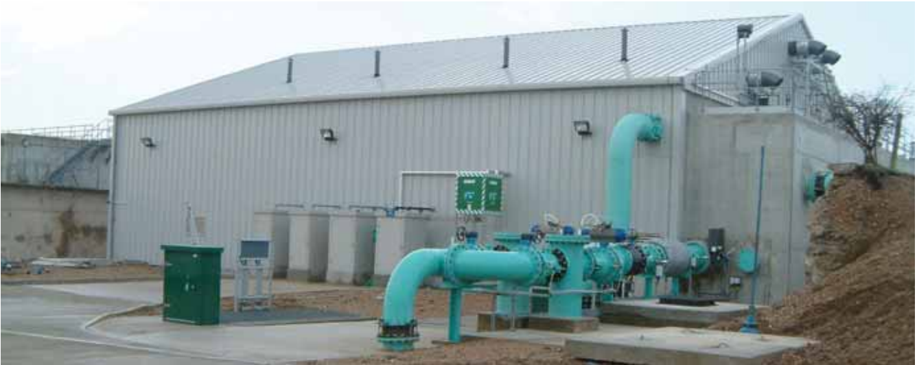
External view of Chertsey Microfiltration Plant
