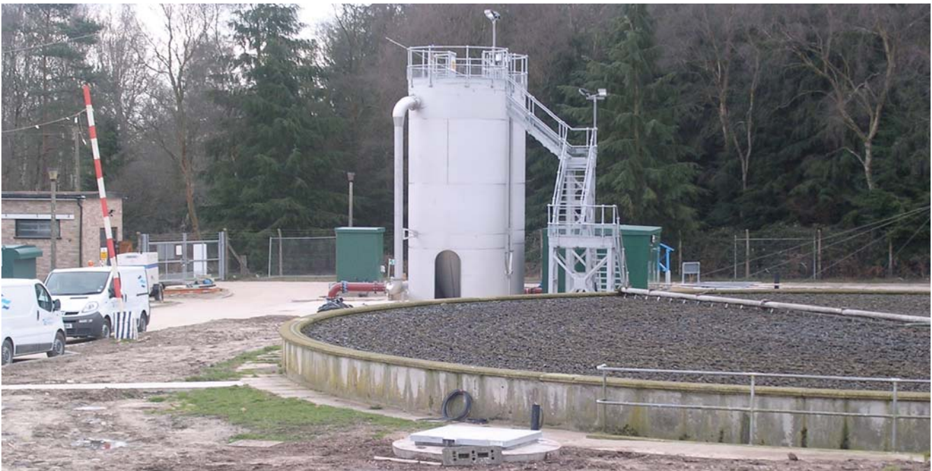
Lyndhurst WTW: Upgrade incorporating chemical dosing & tertiary moving bed sand filters
