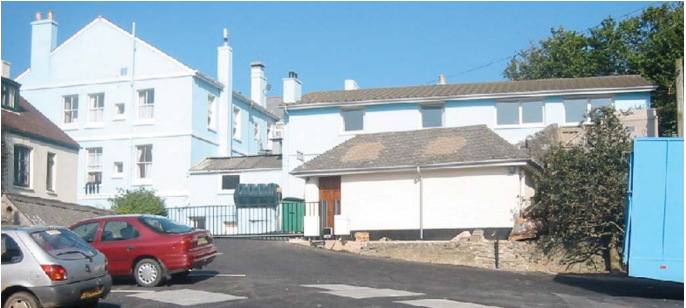
Slapton & Torcross: Torcross pumping station under hotel car park & MCC building is a converted toilet
