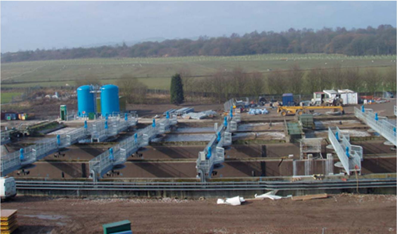
Hyndburn WwTW Quality & maintenance improvements
