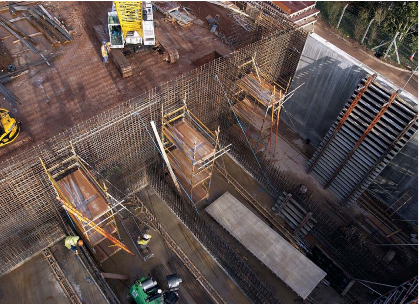
Cumwhinton: WTW under construction
