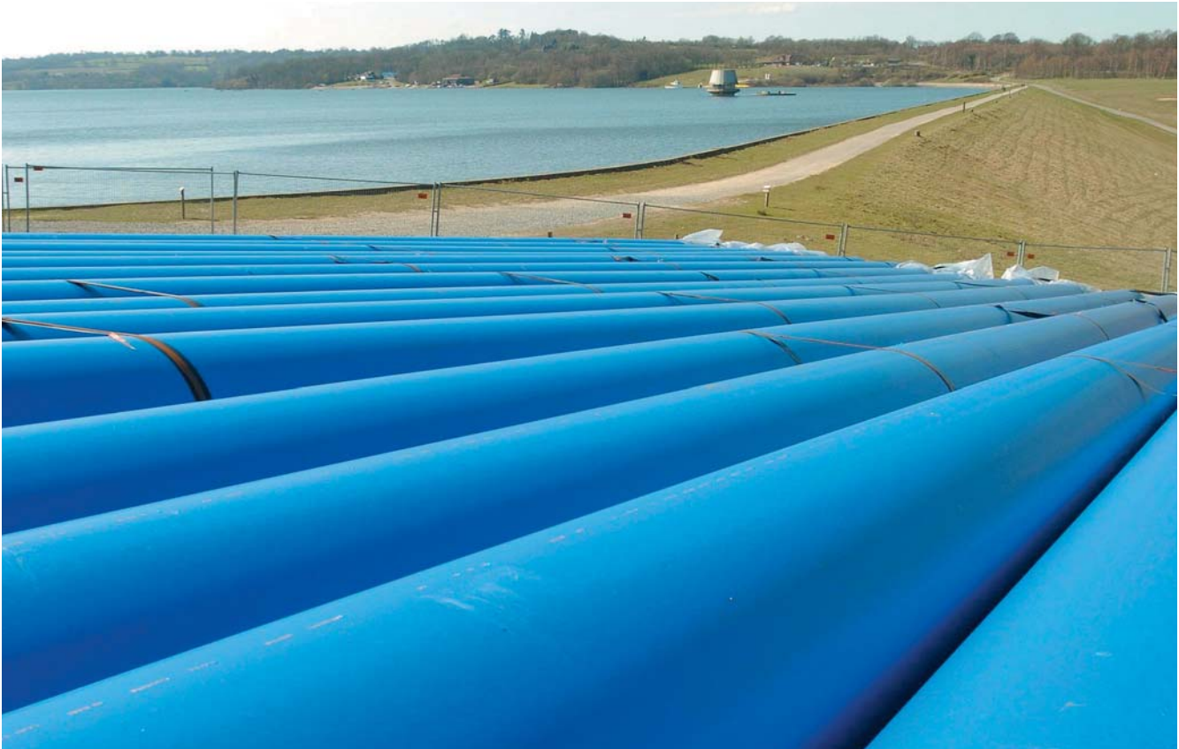
Just some of the 180 pipes required to cross Bewl Reservoir
