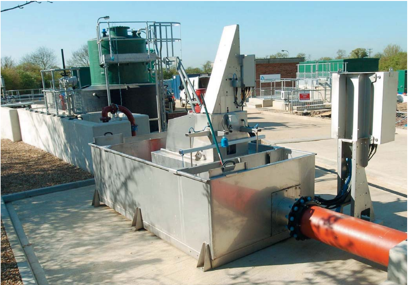
Sutton Valence inlet works
