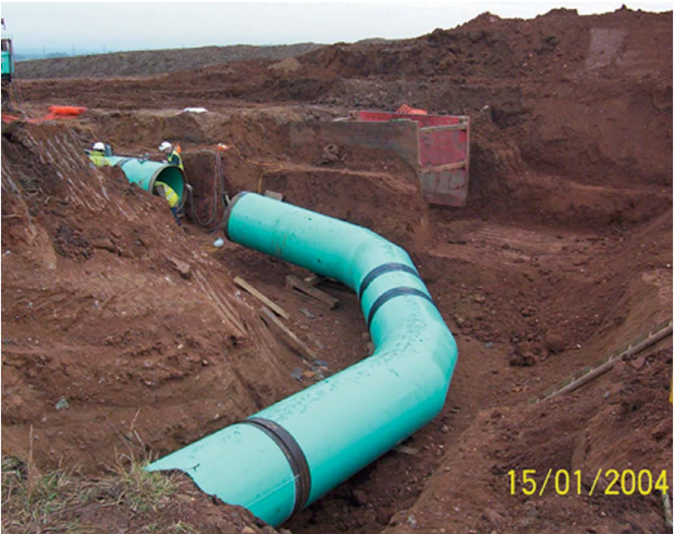
Melbourne WTW: Installation of welded steel pipe
