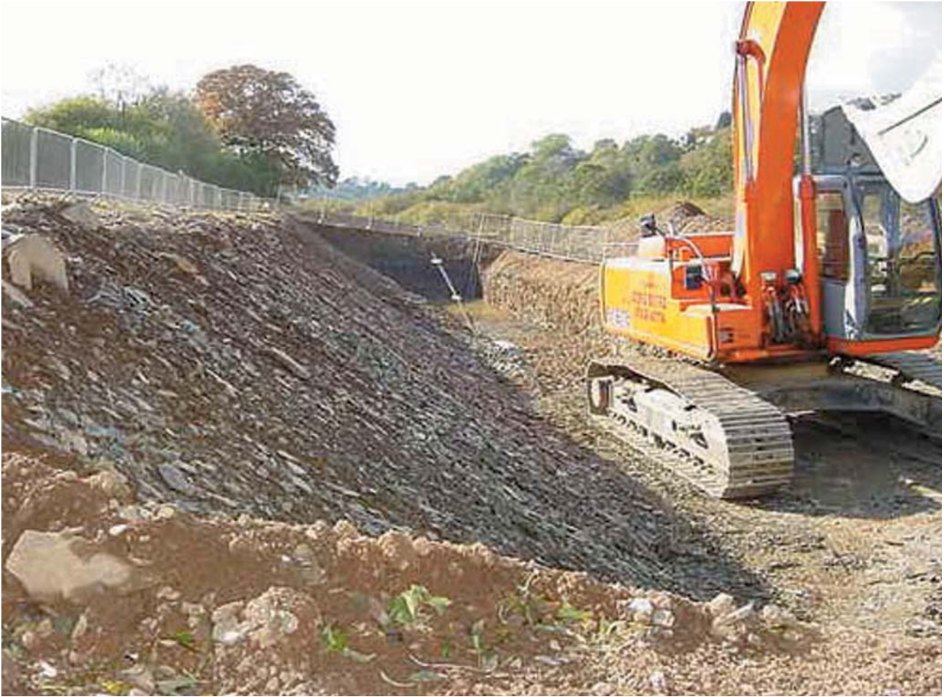
Removal of a DG5 flooding problem at Hayesend Farm
