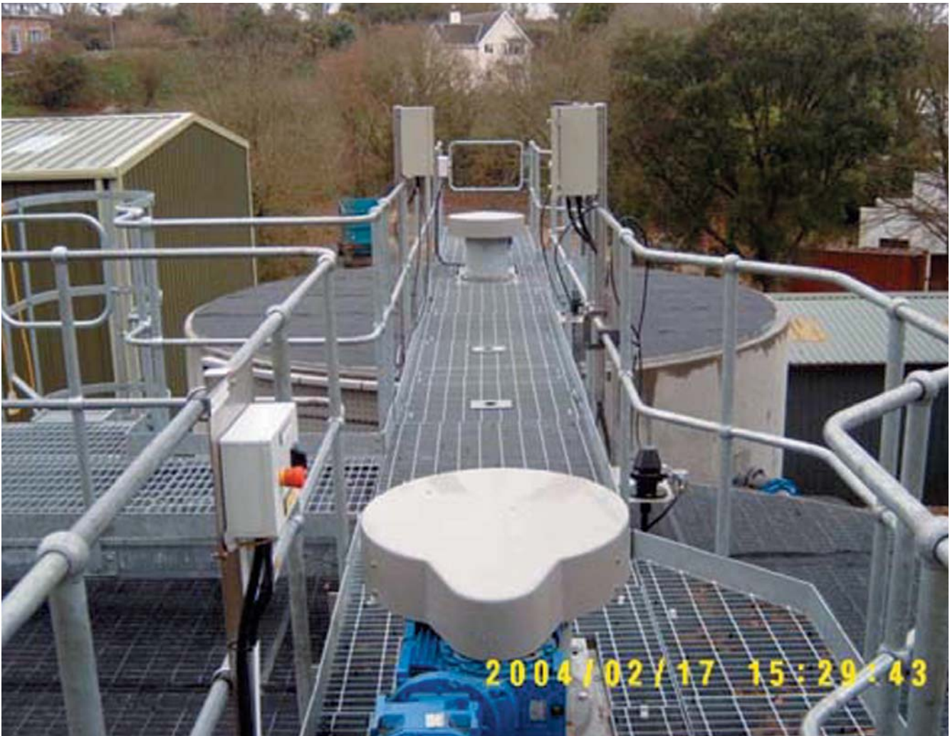
Jersey Washwater Recovery Scheme: Thickener Bridge.
