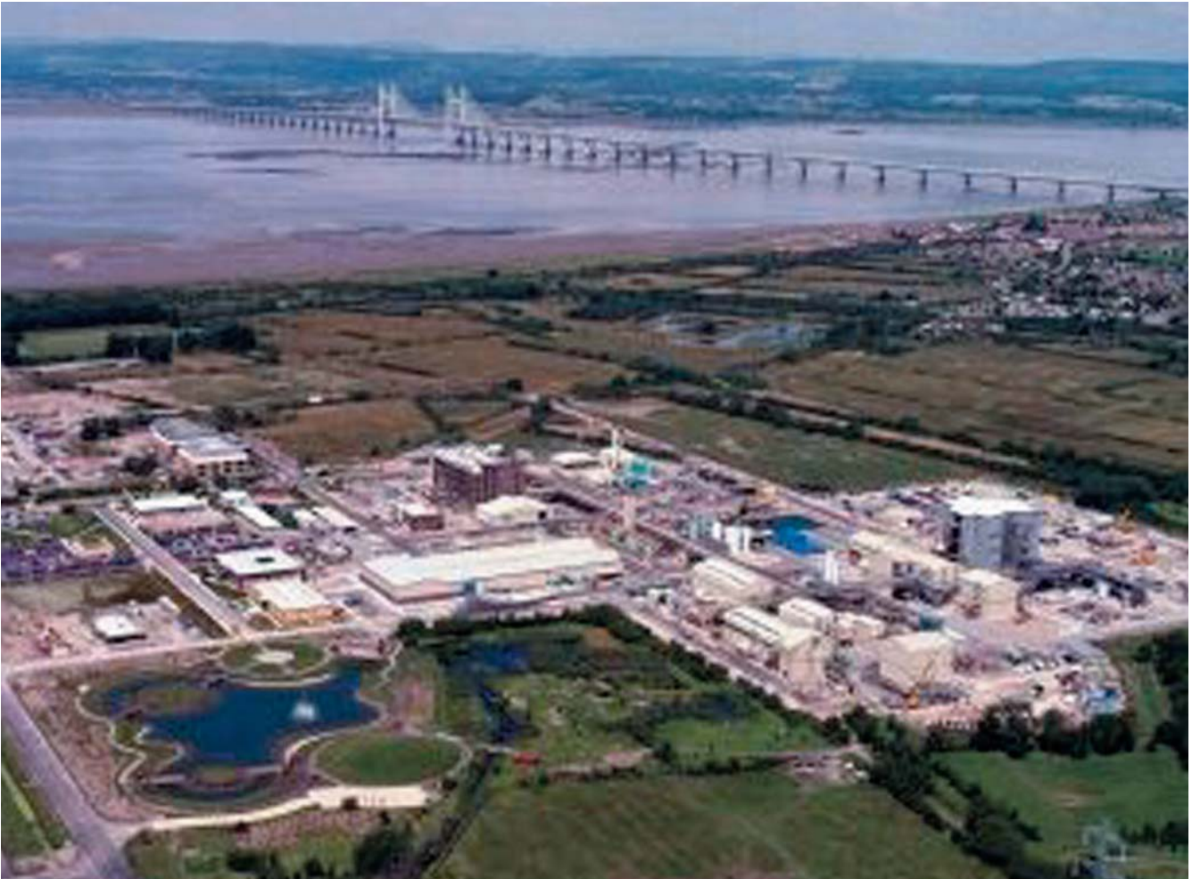
Avlon ETP: Overview of Avlon Works prior to commencement of construction
