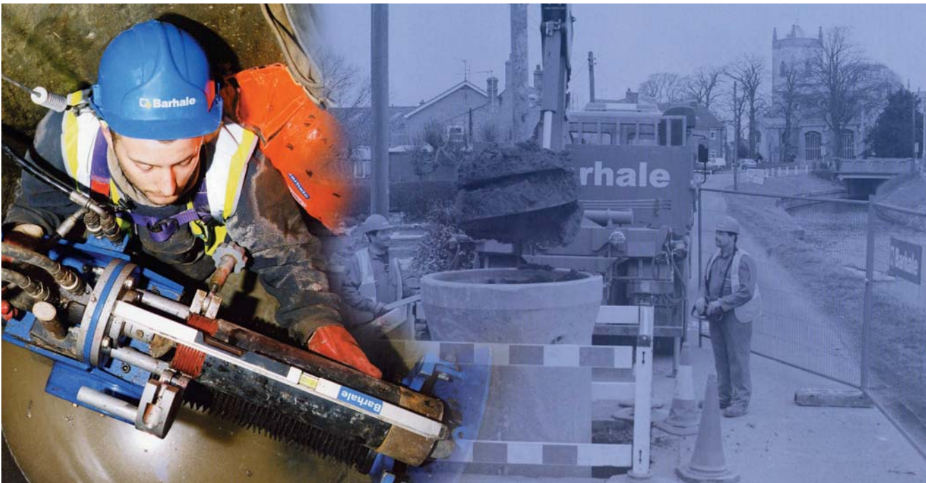
Installing the vacuum sewerage system
