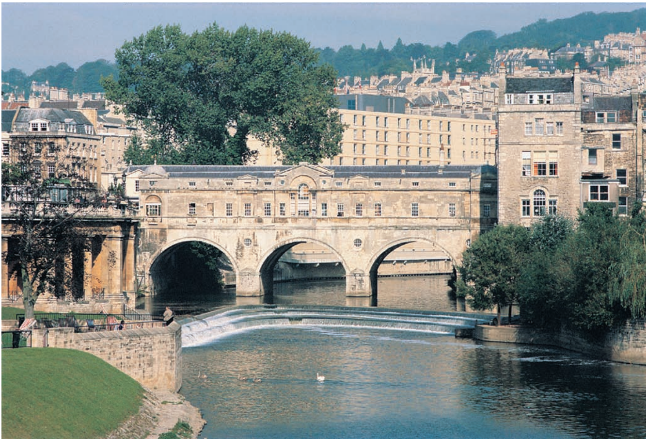
Bath Pultney Bridge (courtesy Wessex Water).
