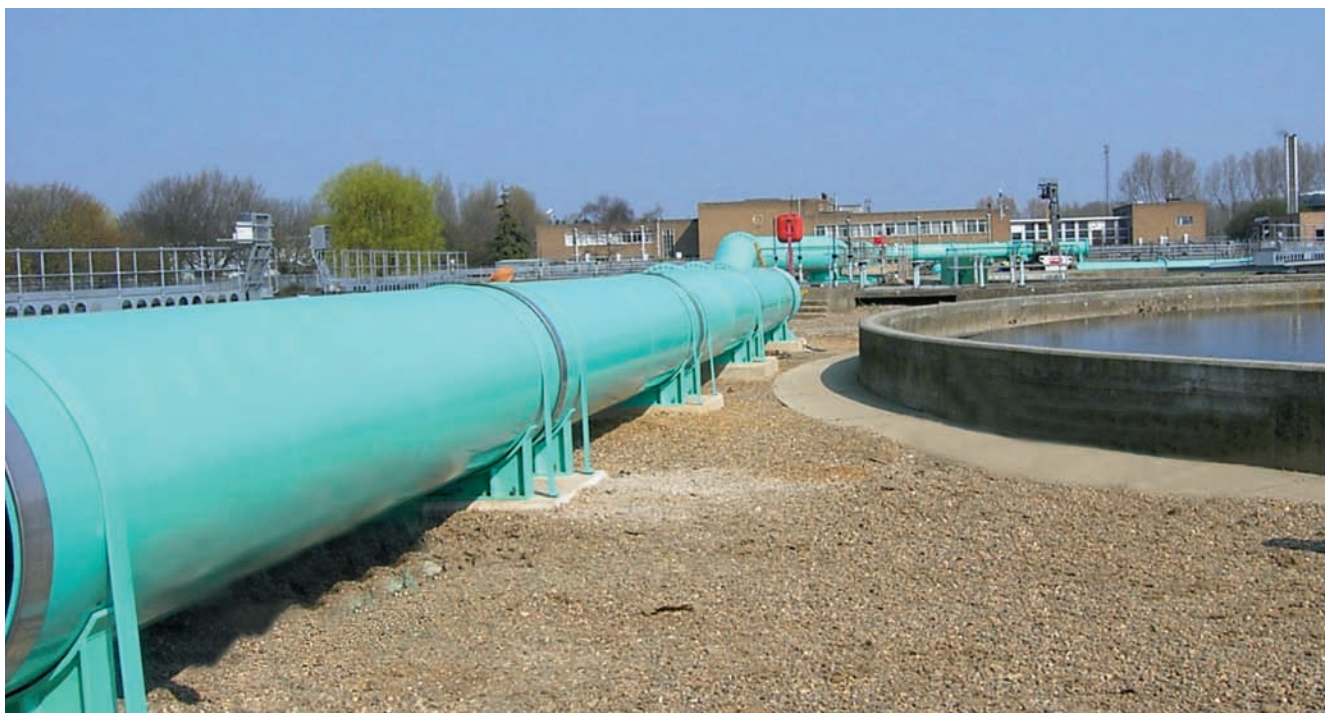
New air distribution mains to existing treatment diffusers (courtesy Thames Water Utilities Ltd).
