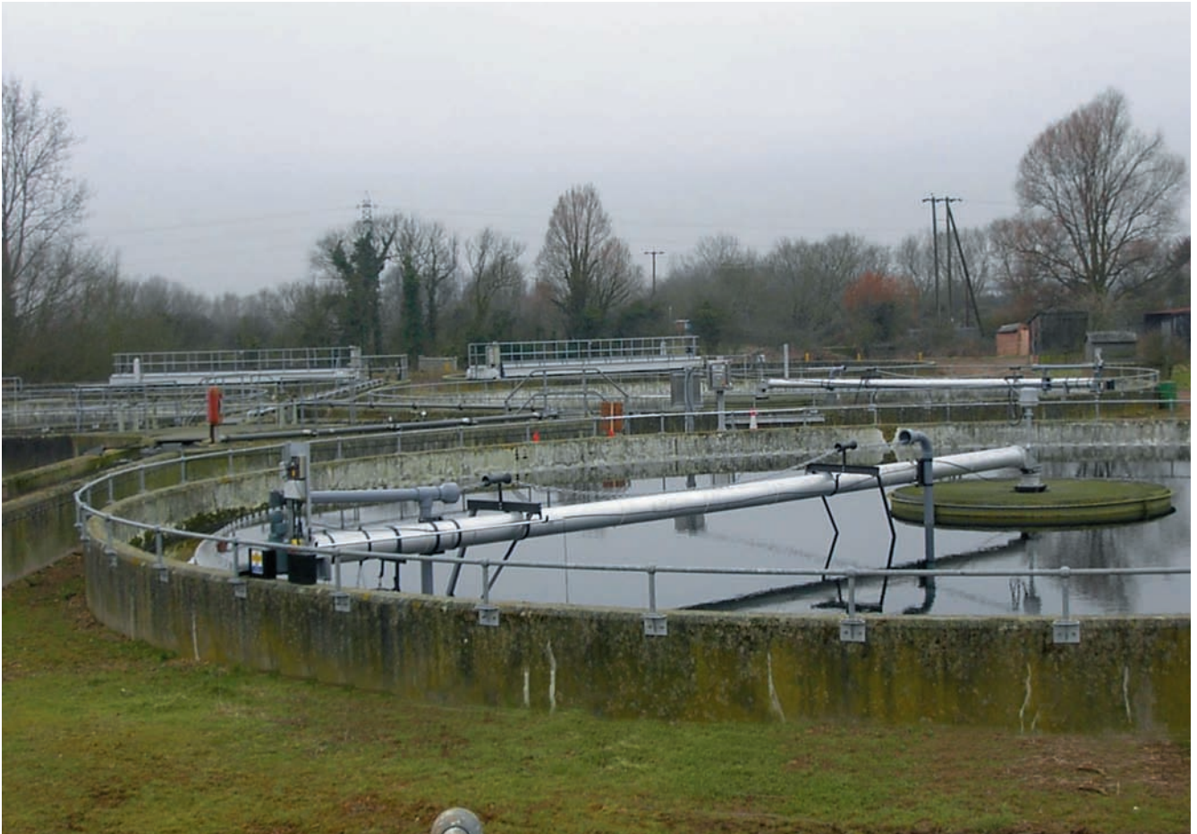
Refurbished final settlement tanks (courtesy Thames Water Utilities Ltd).
