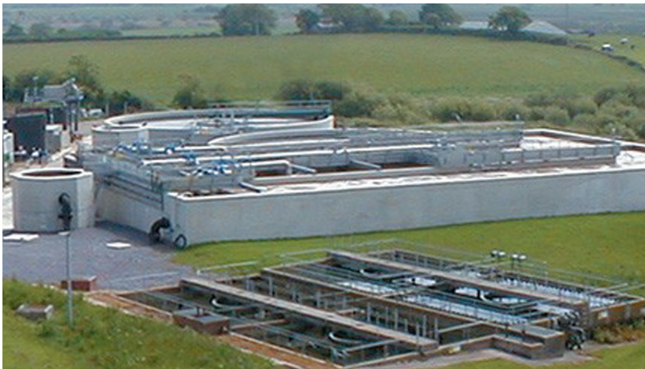
Llangefni WwTW (courtesy Meica Process Limited).
