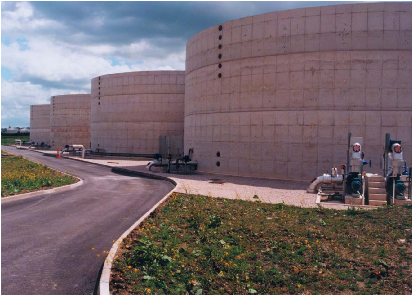
Completed secondary digestion tanks at Warrington (courtesy MWH & United Utilities PLC)
