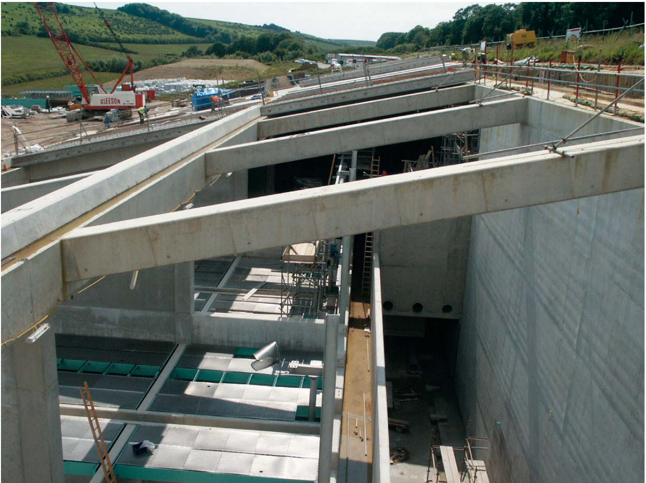
Dover/Folkestone (Broomfield Bank) roof beams over BAFF (courtesy Brightwater Engineering Ltd)
