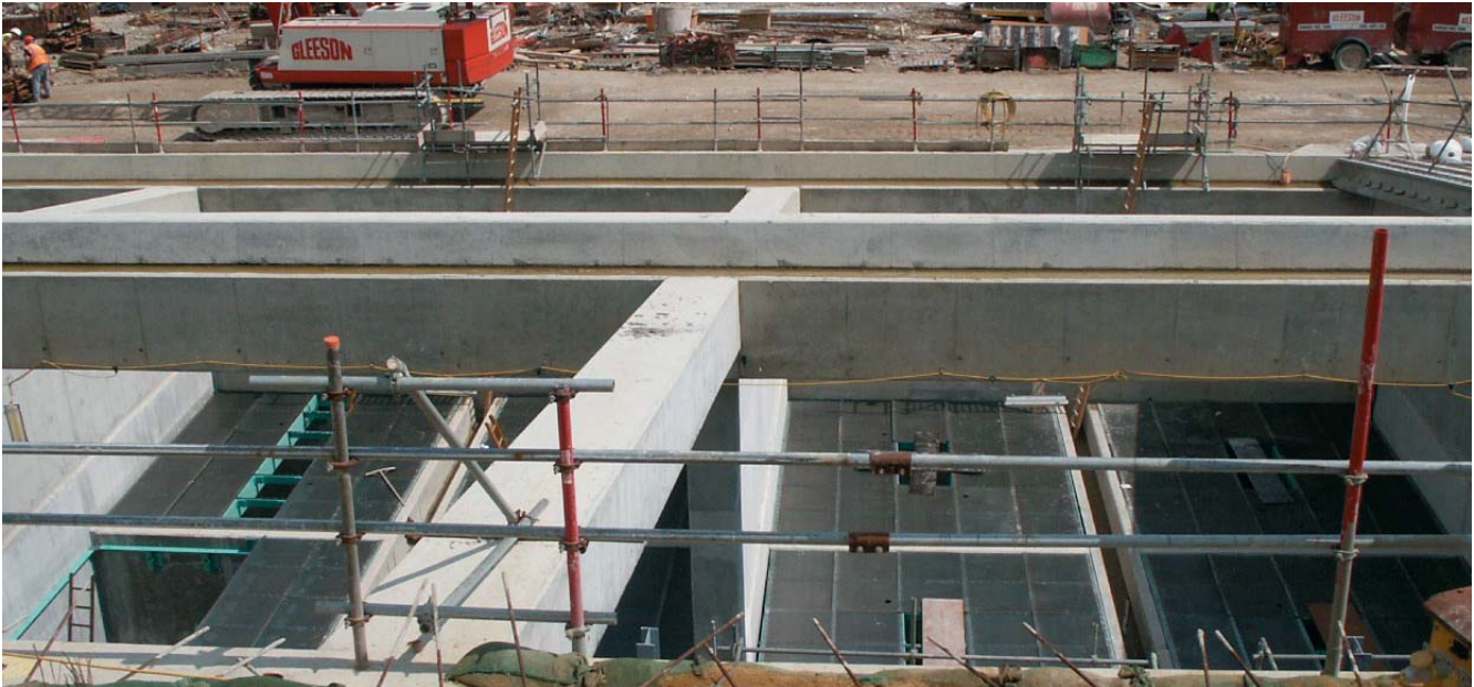
Dover/Folkestone (Broomfield Bank) roof beams over BAFF (courtesy Brightwater Engineering Ltd)
